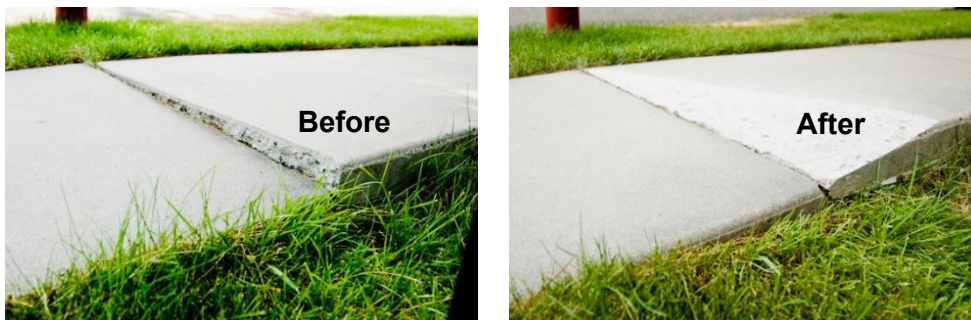
Figure 6: Precision Sidewalk Safety Work Example
